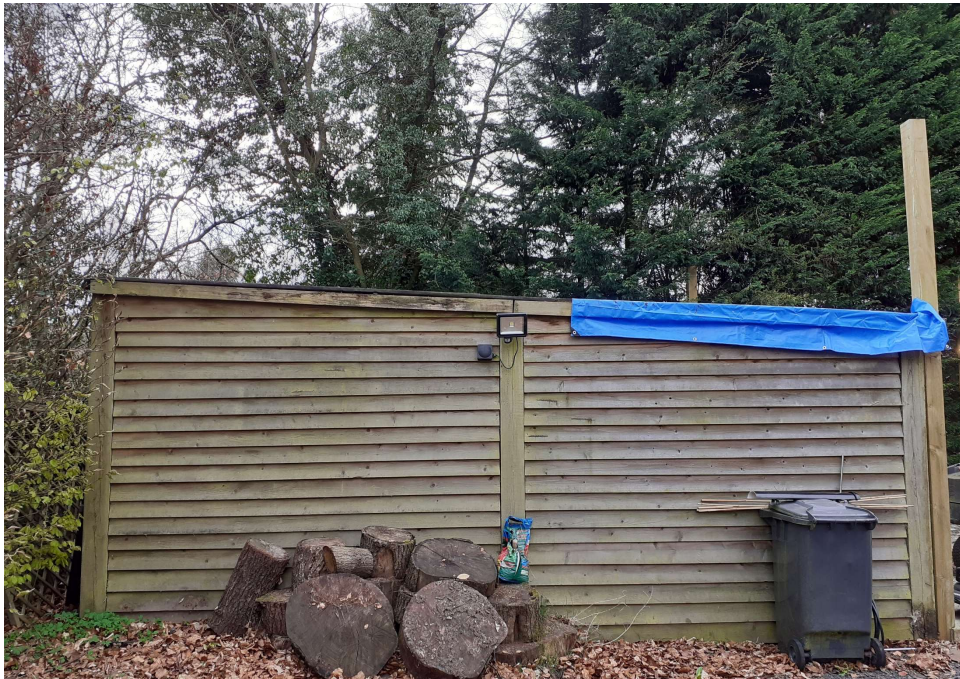
East elevation of existing storage shed
